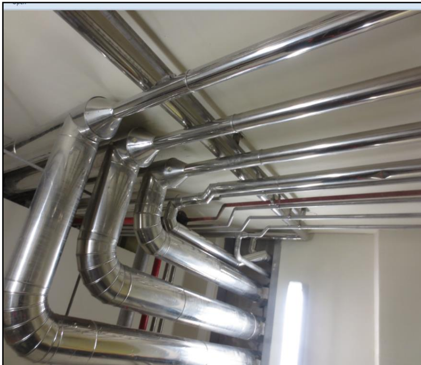
THERMAL ISOLATION INOX IN FOOD-RELATED COMPANY.
