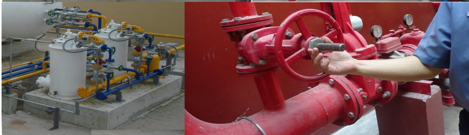
DESIGN- INSTALL FIRE PROTECTION SYSTEM
